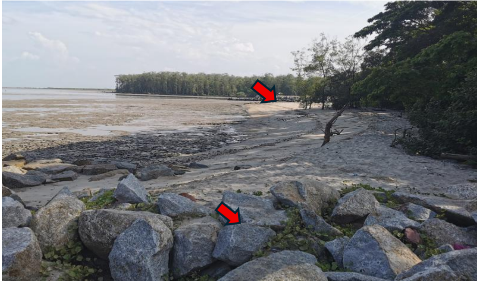
Figure 3.8: Granite groins were placed since 1998 as erosion control and to stabilize the shoreline south from Teluk Malas (Red arrows).
