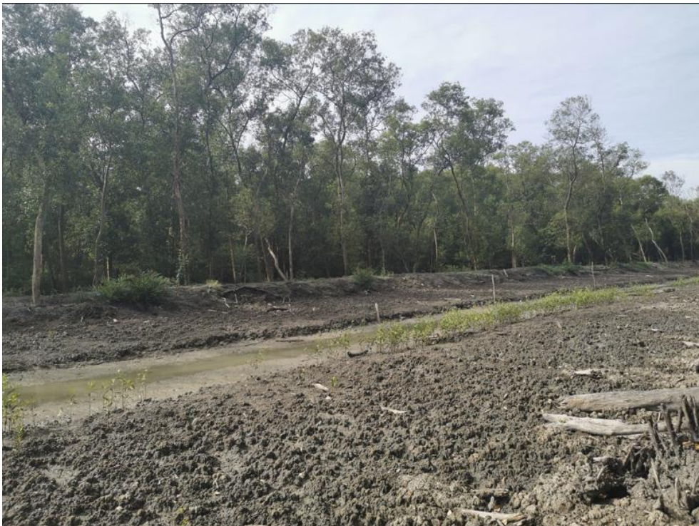
Figure 3.51: A canal with width 30+ meters and length 500+ meters at Encroachment Site A (5° 30' 33.64" N, 100° 22' 30.83" E). Photo dated March 2025
